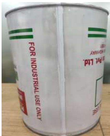
Touch-up Paint Applied weld seam
